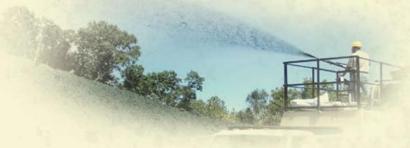
HydraMatriCx<sup>™</sup> Series high-performance hydraulic erosion control products are made with a proprietary blend of straw, reclaimed cotton plant material, tackifiers, and polymers.
